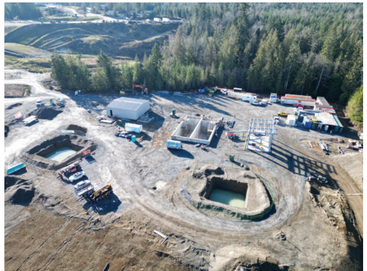
New Wastewater Treatment Plant Construction
