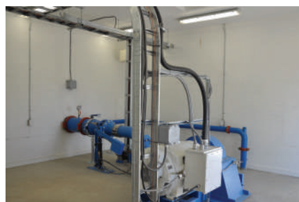
Micro Hydro Project turbine and generator
