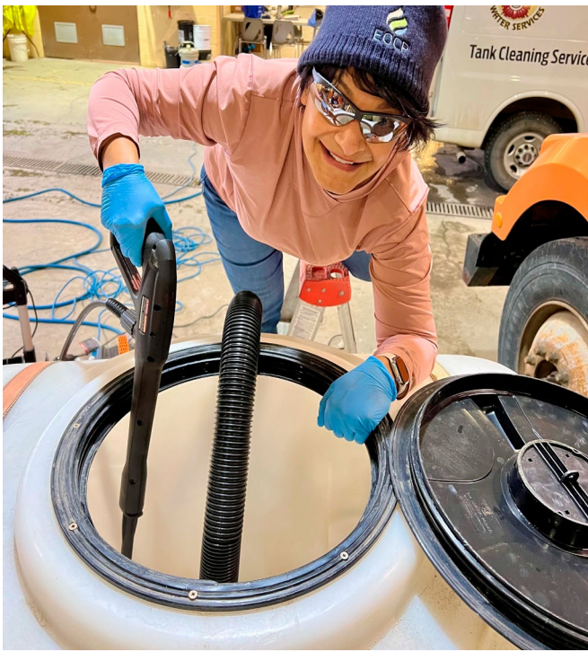
Kalpna (EOCP's President and CEO) pressure-washing a water tank
