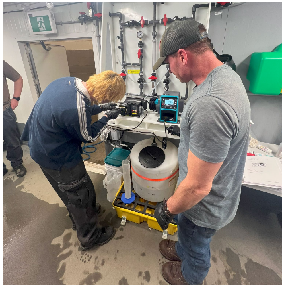
Alex (Engineering student) and Aaron (Operator) doing maintenance work on the sodium hypochlorite pump
