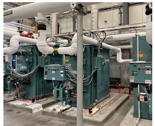
Boilers to Heat the Water in the Winter
