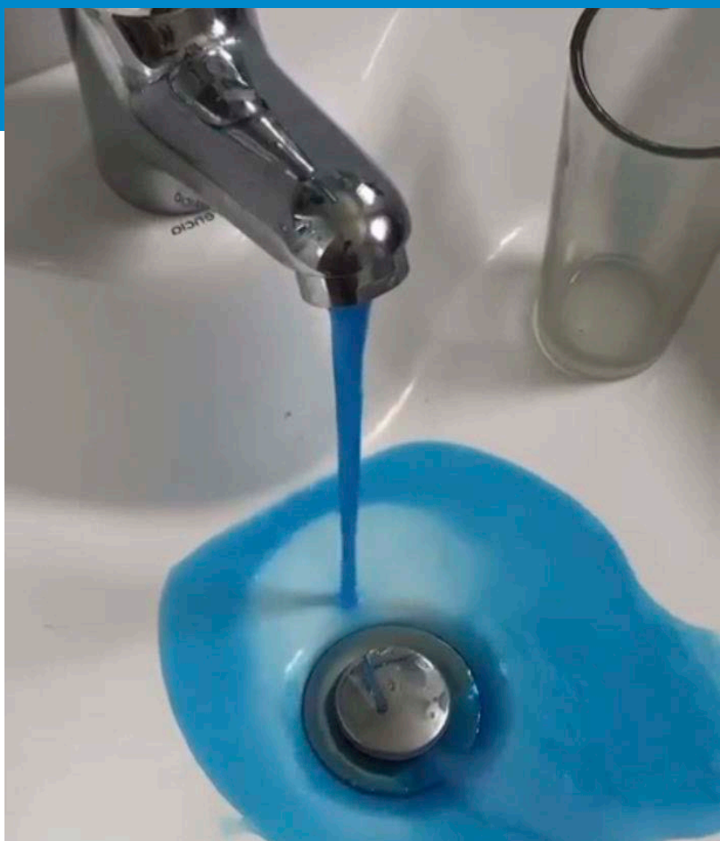
Figure 2: Acid Blue 9, used for algae control backflowed into the building's drinking water system from a building's air conditioning system
