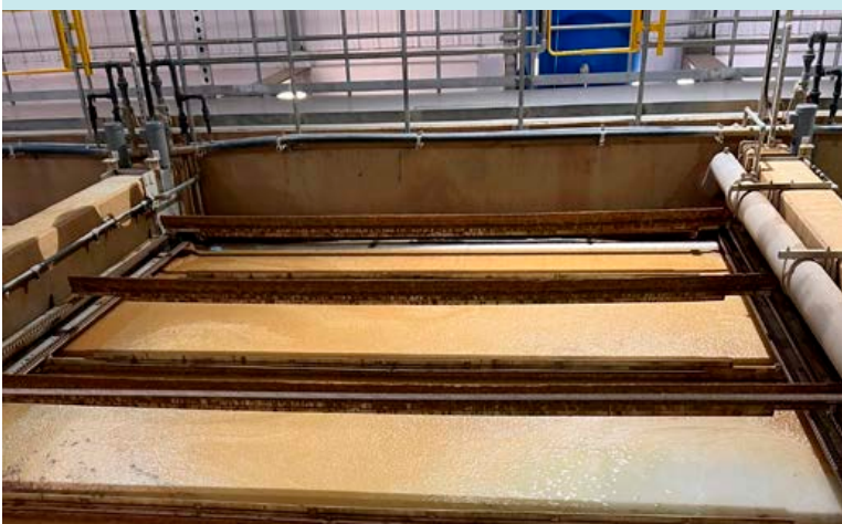
Combined DAF and filtration basin at Powers Creek
