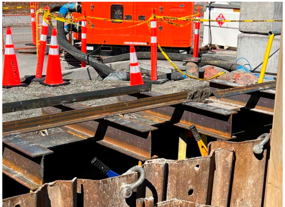
Sheet piles in foreground to enable dewatering for manhole replacement, I-beam and cradles behind to prevent BC Hydro vault from subsiding
