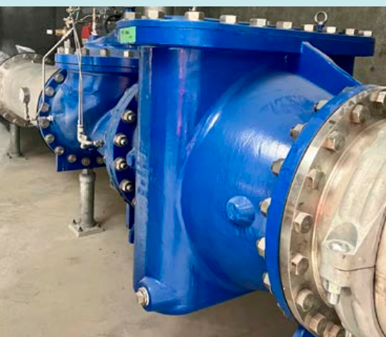
Coarse screen and PRV
