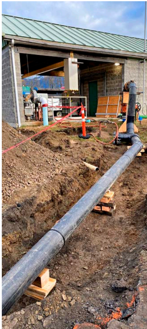
Completed emergency bypass
