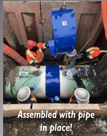
A permanent repair complete!
