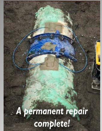
Assembled with pipe in place!
