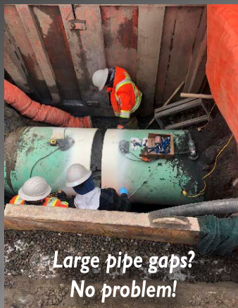
Watermain leak exposed
