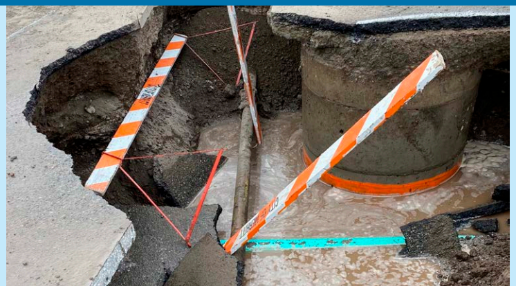
Coldwater Avenue sinkhole exposed a gas line which needed to be supported
