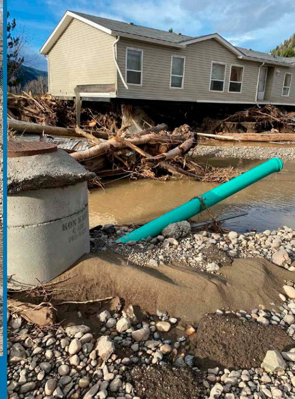
Pine Street washout exposing wastewater collection system
