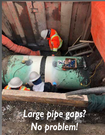
Watermain leak exposed
