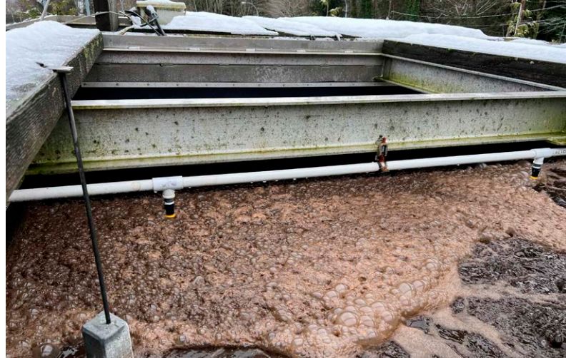
▲ Sprinkler System Above Aeration Tank
