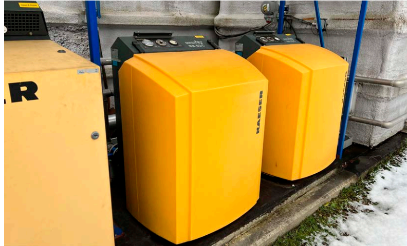
▲ Process Blowers (Aeration, Equalization, Sludge Holding and Membrane Bio-reactor Tanks)
