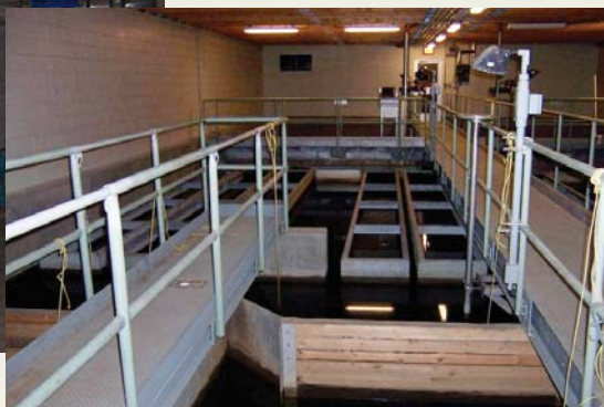
Flocculation-Sedimentation-Filtration Area
