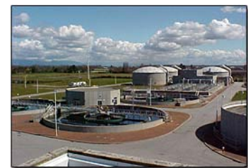
Clarifiers and Trickling Filters
