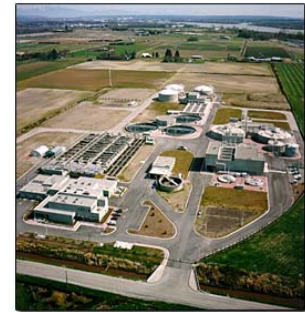
Lulu Island WWTP
