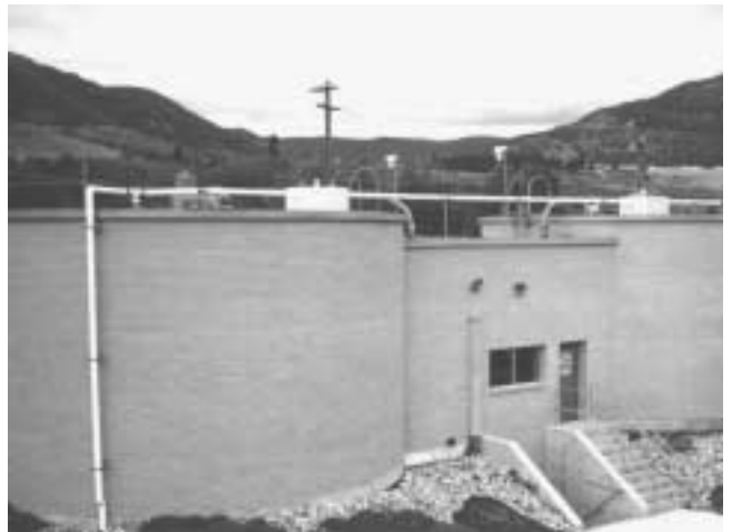
Fermenters with overhead odor line that runs to primary's.
