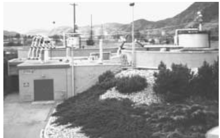
The City of Penticton Advanced Wastewater Treatment Plant was constructed in 1990. It is a Class IV plant that presently treats flows of 15,000 m 3 per day. The treatment process includes tertiary treatment, sludge composting, disinfection and effluent irrigation. (Plant profile continued on page 6).
