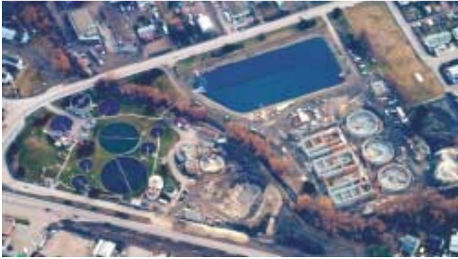
The existing wastewater plant is on the left with the new construction on the right.
