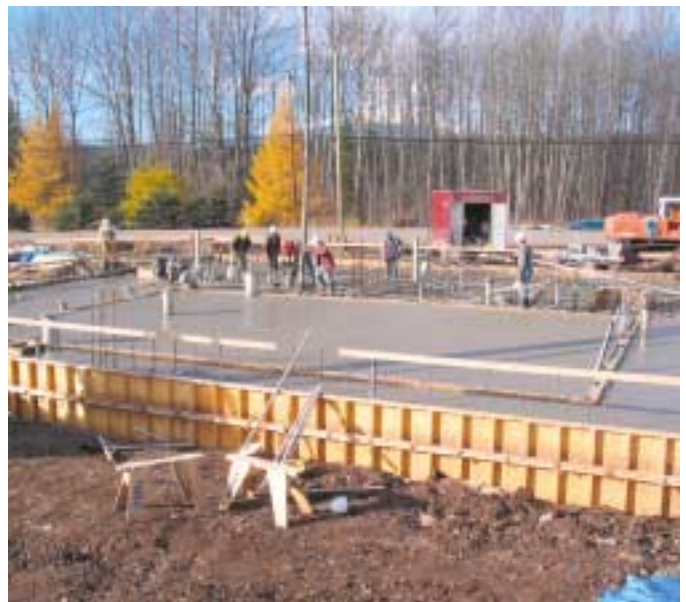
Telkwa Water Treatment Plant Construction
