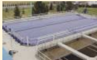
The photo above shows the new primary tank covers at the Kelowna Wastewater Treatment Plant. The odor control covers were designed by the two operators shown right – Vince Hughes and Mike Humes.
