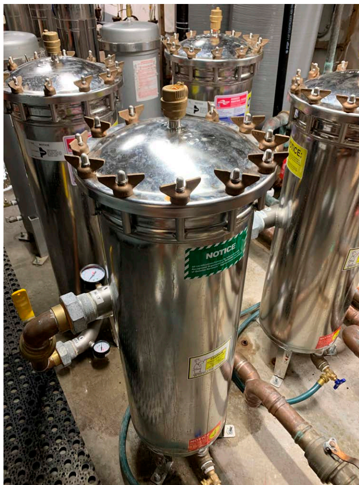
Filters In Series Going From 10 \mu\text{m} to 5 \mu\text{m} to 1 \mu\text{m} to 0.35 \mu\text{m} .
