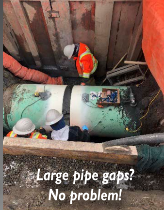
Watermain leak exposed
