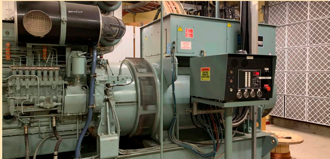
Generator to provide back-up power for pumps
