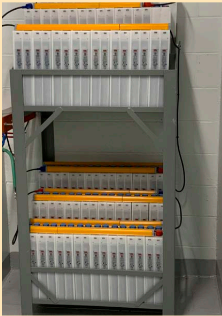
Battery packs to provide back-up power for electronics
