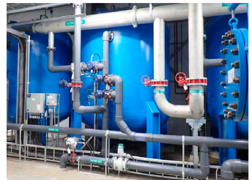
Bayoxide E33 Vessels for Arsenic Adsorption
