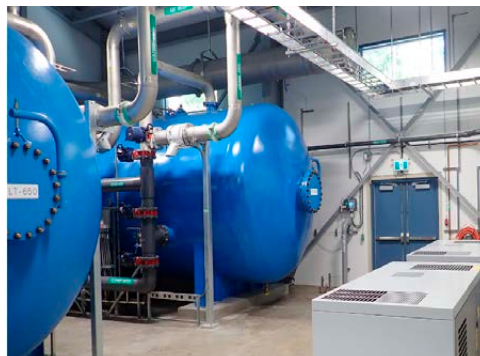
Greensand Plus Filters for Manganese Removal
