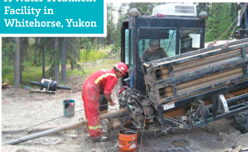
Horizontal drilling of water intake pipe.
