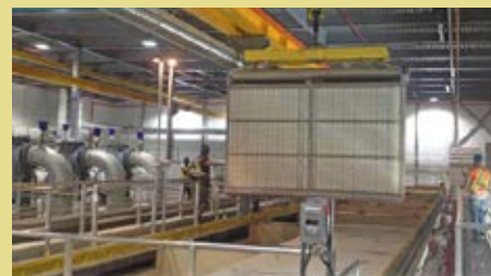
7 Primary and secondary membrane filters being installed. They remove .1 micron particulates and protozoa, including Cryptosporidium and Giardia .
