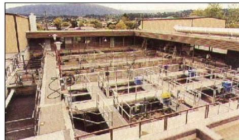
In the solids contact tanks the suspended excess biomass is flocculated and aerated by the Turborators. Additional soluble carbon food substrates are also utilized by the biomass.
